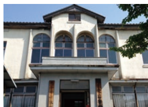
Nagahama City, Shiga Prefecture: Kohoku Library
